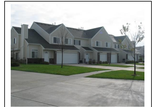
Example of Single-Family Attached
