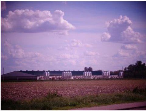
Example of an Animal Confinement Building
