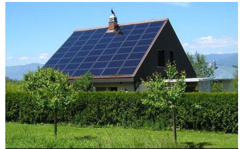
Example of a Solar Conversion System, Structure-mounted
