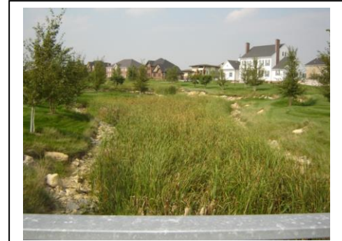
Example of a Drainageway or Surface Drain
